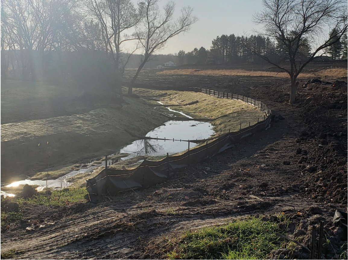
View looking SE at channel after unpermitted activity. Appears silt fence is placed perpendicular to the channel damming the water flow. 11.5.2020
