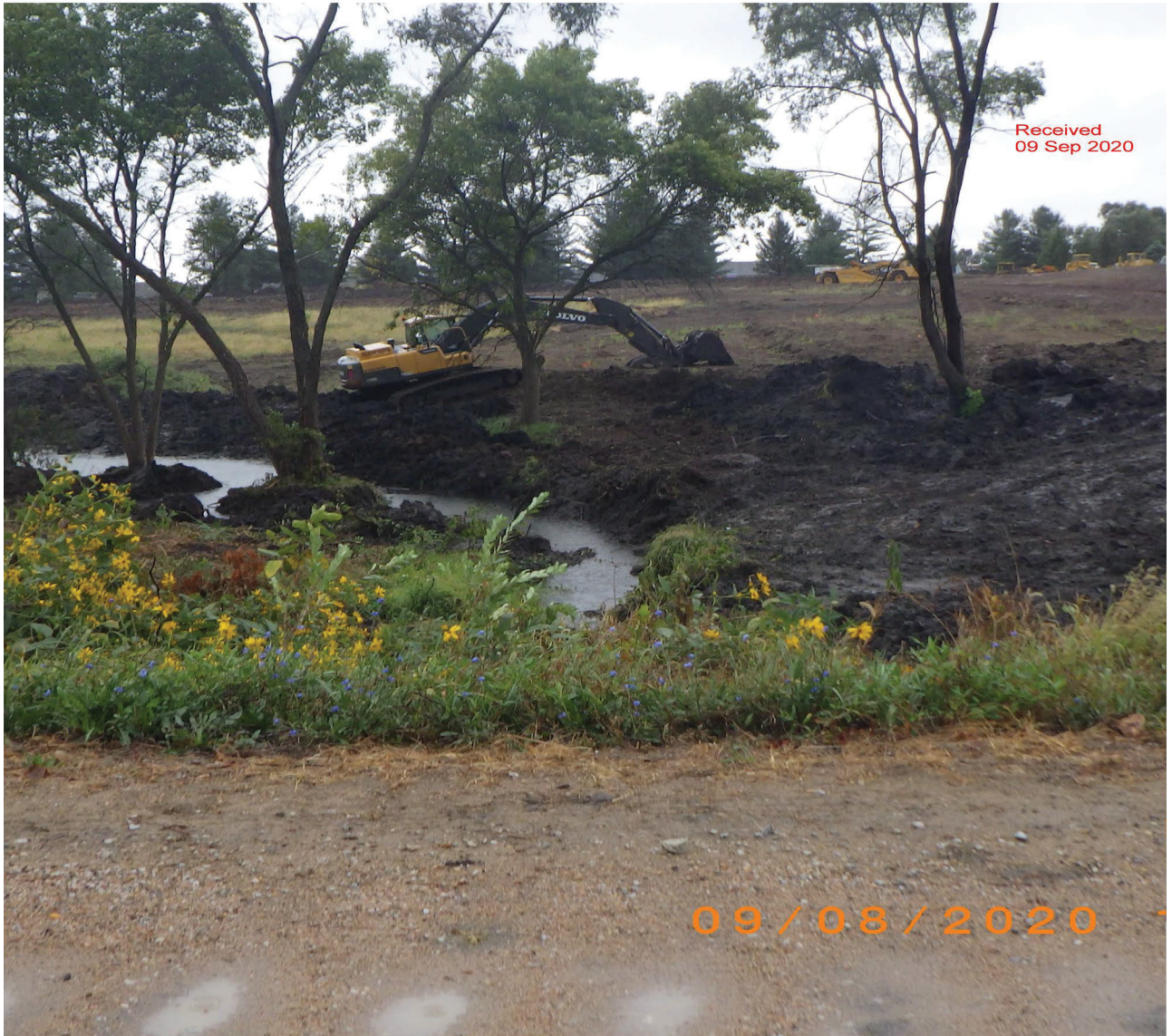
Photo provided by my anonymous neighbor reporting violation looking south from Bennet Road. This photo shows no BMPs and working being conducted along the channel. It appears there is fill material placed on both sides of the channel. 9.8.2020
